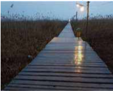
Figure 14. Wooden Bridge on the Bandar-e-Kiashahr Lagoon
