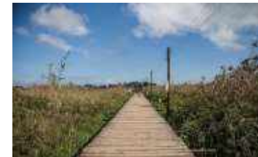
Image I.2-4: Wooden Bridge in Bandar-e-Kiashahr
